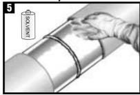
Ensure that the mainline coating edges are beveled to 30° minimum. If there is the presence of oil, grease, or other surface contaminants; clean the exposed steel and adjacent pipe coating with an approved solvent cleanser.
