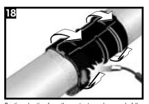
Continue heating from the centre toward one end of the sleeve until recovery is complete. In a similar manner, heat and shrink the remaining side.
