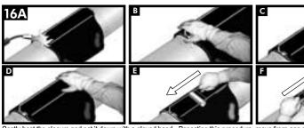
Gently heat the closure and pat it down with a gloved hand. Repeating this procedure, move from one side to the other. Smooth any wrinkles by gently working them outward from the centre of the closure with a roller.
