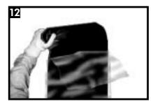
Partially remove the release liner [approximately 1 metre (3') from the edge] from the corner trimmed sleeve edge.
