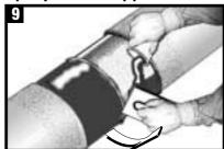
Apply mixed epoxy to a uniform specified thickness of 4-6 mils (100-150 microns) on all exposed bare metal plus 10mm (0.5") onto the adjacent pipe coating using the applicator pads as supplied or an approved tool. Do not apply the epoxy to the mainline coating.
